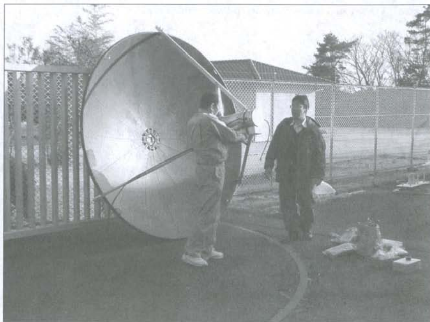
Fig. 4 Primary Feed for 23 cm
