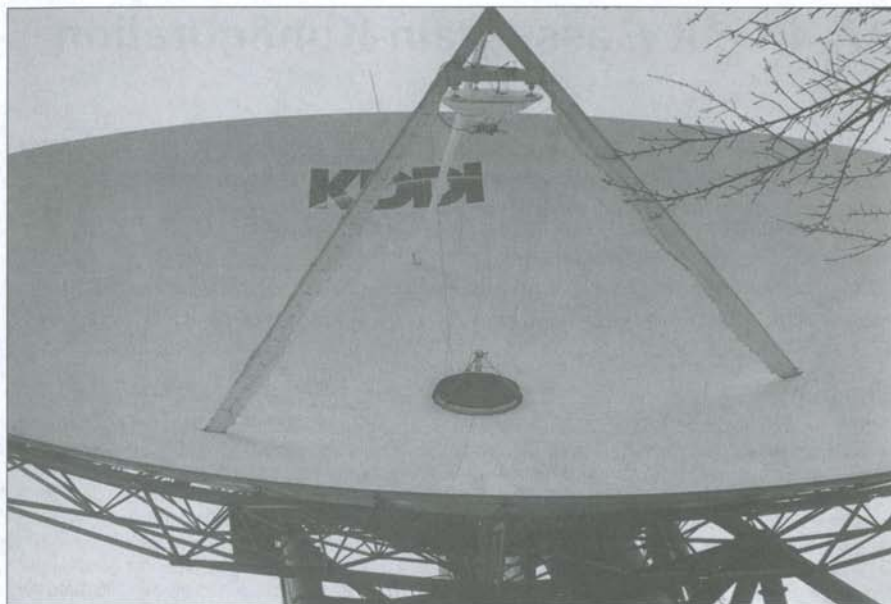
Fig. 15 KDDI Antenna Equipped with 2m, 70cm and 23cm Feeds
