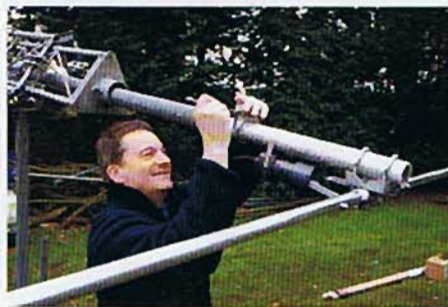
PHOTO 4: A trailer-mounted Versatower was used for the Dual Beam Pro.
